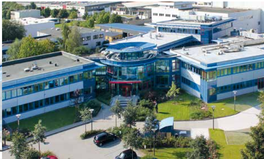
Stern Technology Center in Ahrensburg, near Hamburg
